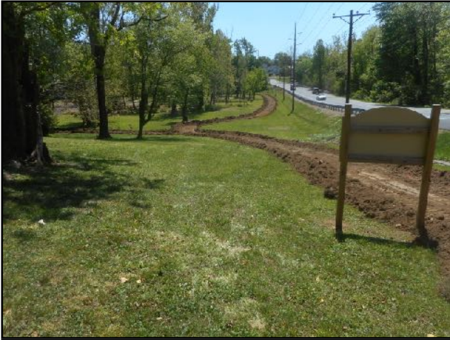
Eight foot wide path created, bulldozing 8 inches deep.
