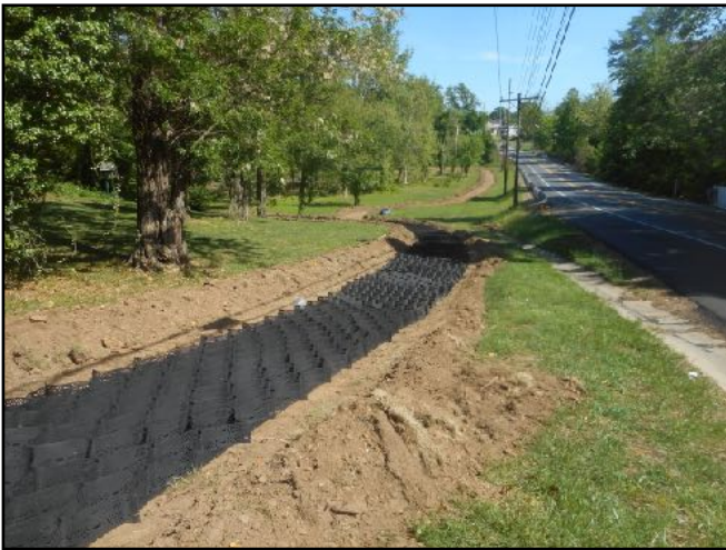
Geo-grid placed to be filled with stones as foundation for the path.
