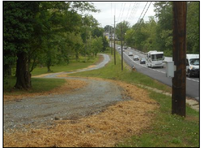
Final layers and grading completed along the same section. Straw and grass seed will fill in the lawn up to the trail edges.
