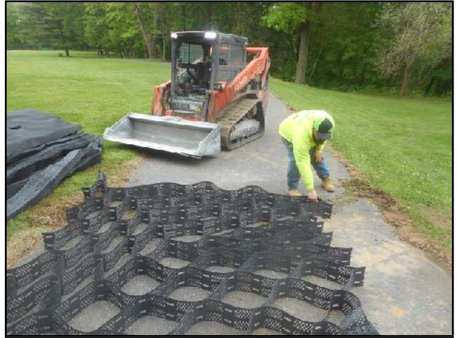
A close-up of the 6" tall plastic geo-grid, before being filled with gravel.
